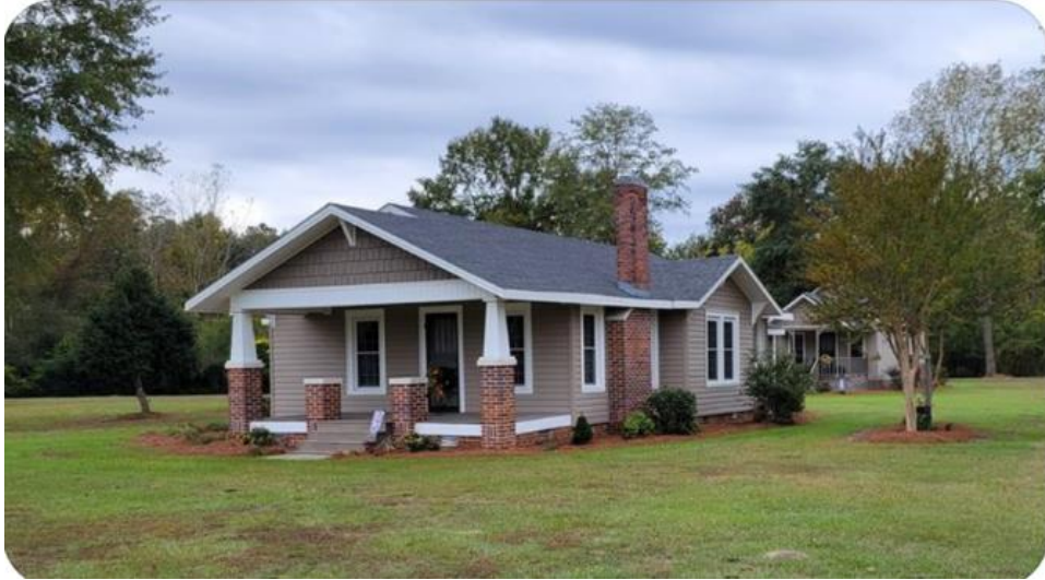
Restored Post Office
