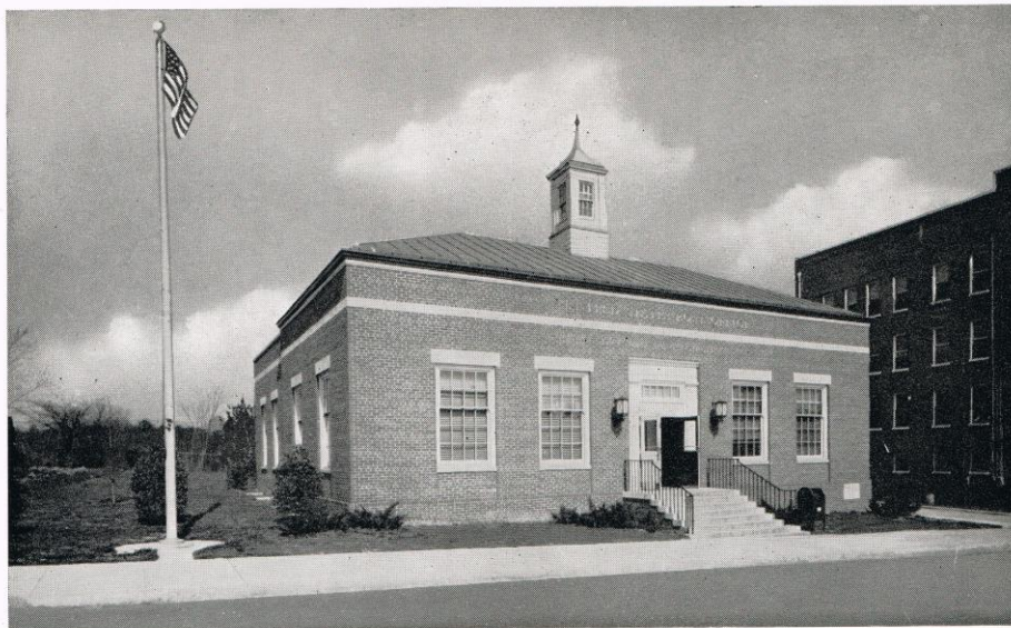
United States Post Office, Leaksville, North Carolina
